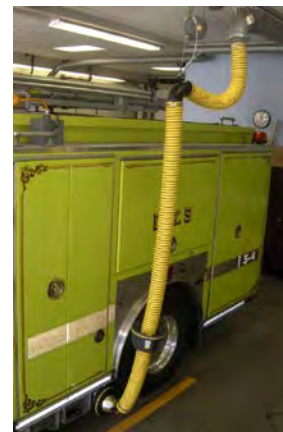
Plymovent System hooked up to an existing Nederman rail
